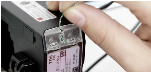
Once the terminal cover has been placed, the transformer sealed.
